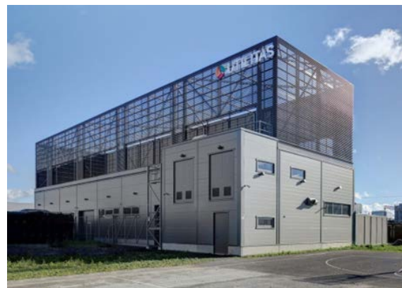
Utilitas' new cooling station
